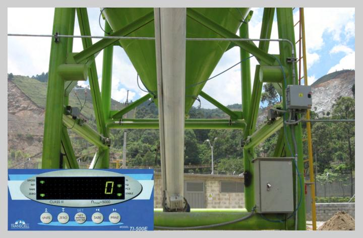
**SiloWeigh Basic** tells you the contents of any silo, feed bin, tank or storage vessel. Better than silo level measurement, SiloWeigh Basic measures the actual silo weight to give a true picture of the quantity on hand.
