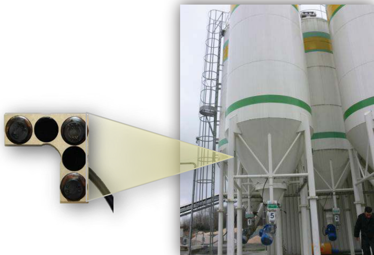
Installation of sensors on round silo legs using weld tabs
